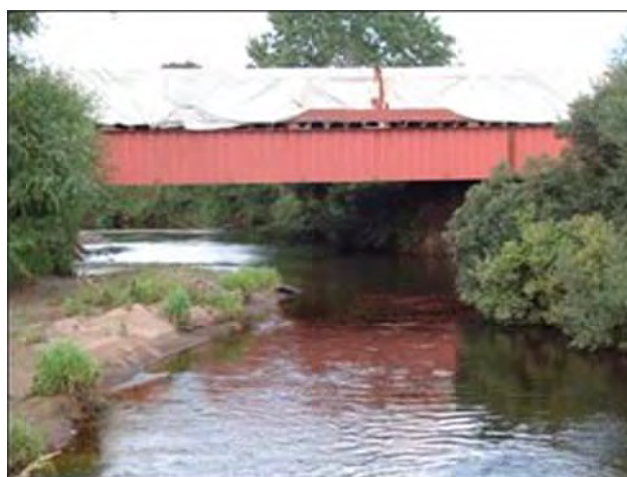
A clear span temporary crossing capable of carrying heavy axle loadings and long wheel base vehicles.
