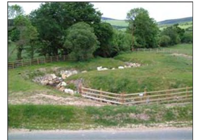
Extreme meanders installed during excavation of a new channel to overcome excessive gradient between the original course of the stream (in the background at tree line) and the point of entry of the newly created channel to a culvert (in foreground under the timber fencing). In this instance there was inadequate provision at the planning and design stage for the necessary land take.
