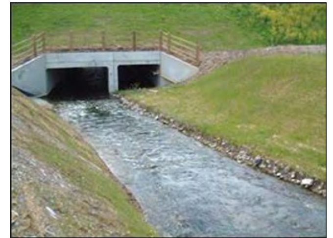
Looking from upstream towards a culvert arrangement. Moderate and flood flows are conveyed in the right hand culvert. Entry to that culvert is dictated by the invert and contour of the right hand portion of the newly created river channel. The left hand bank finished batter angle is approx. 45°. The first portion of the right hand bank to convey the moderate flow is battered to approx. 30°. The extreme right bank area is battered to approx. 45° to convey flood flows.
